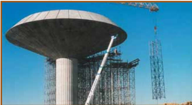
9 th Place / Photographer: J Jung Murray & Roberts: Lanseria 20ML Reservoir and 1.2ML Water Tower
